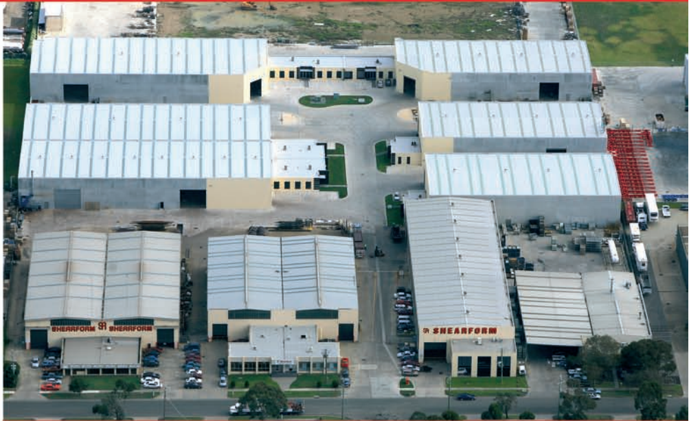
Steel Sales and Service Centre, Dandenong Victoria
